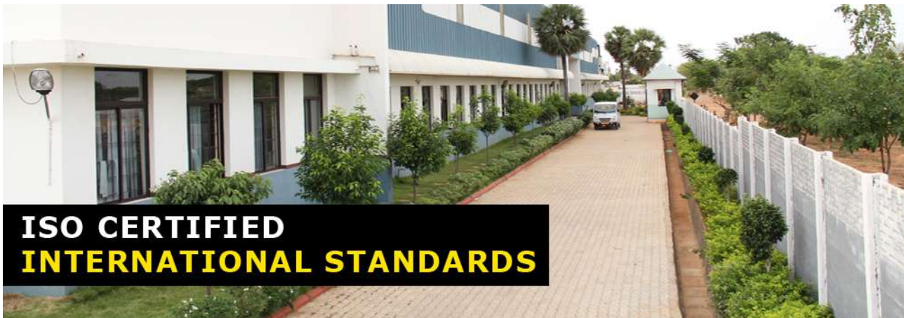
Pipe Hangers & Supports Private Limited - Thanjavur (Land - 112,500 Sq ft & covered shed 40,000 Sq ft)
